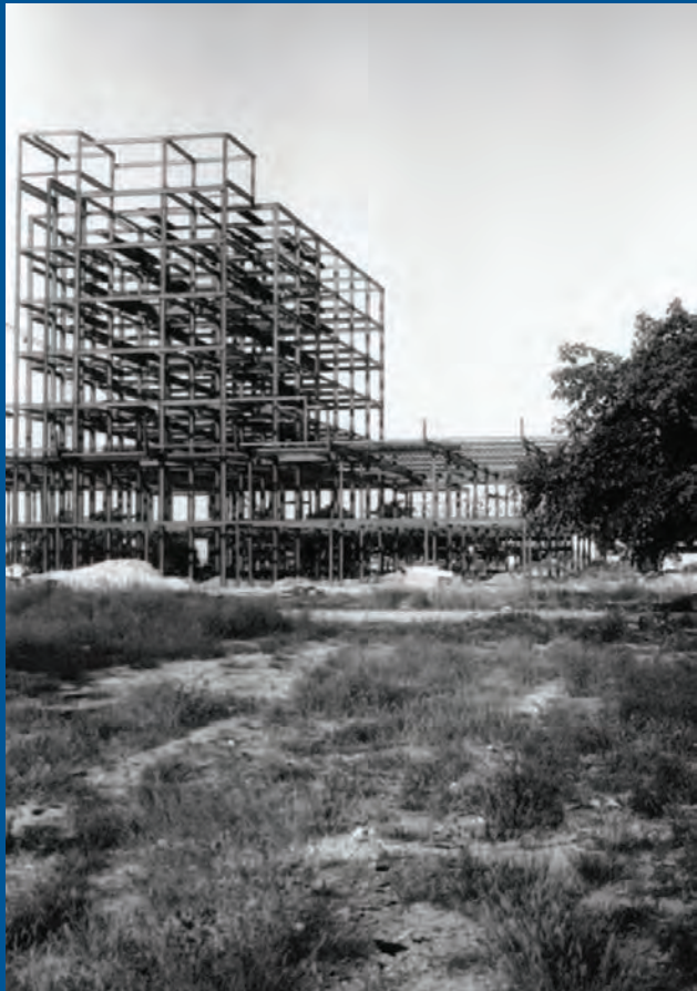
20th Street Terminal under construction - 1957
